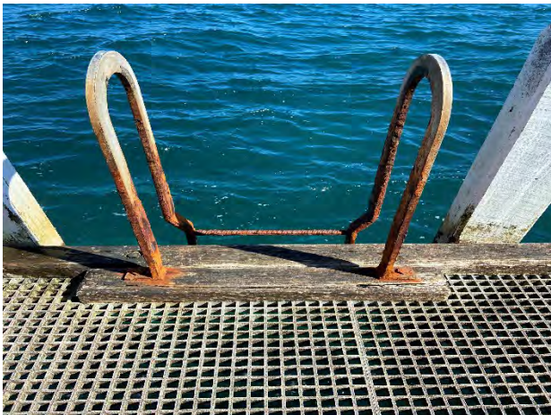
Figure 4-16: General condition of ladders atop main jetty and installed to lower landing
