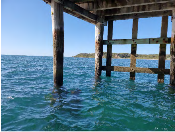
Figure 4-14: New timber walers and fenders at jetty head (left) and older members remaining (right)
