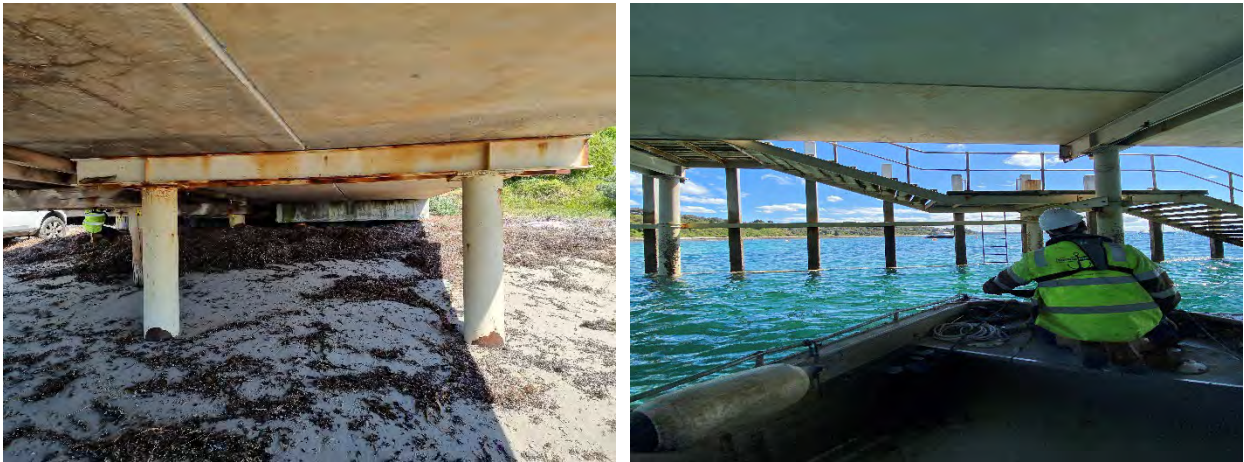
Figure 4-24: General condition of concrete deck soffit
