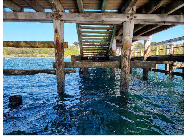
Figure 4-14: New timber walers and fenders at jetty head (left) and older members remaining (right)
