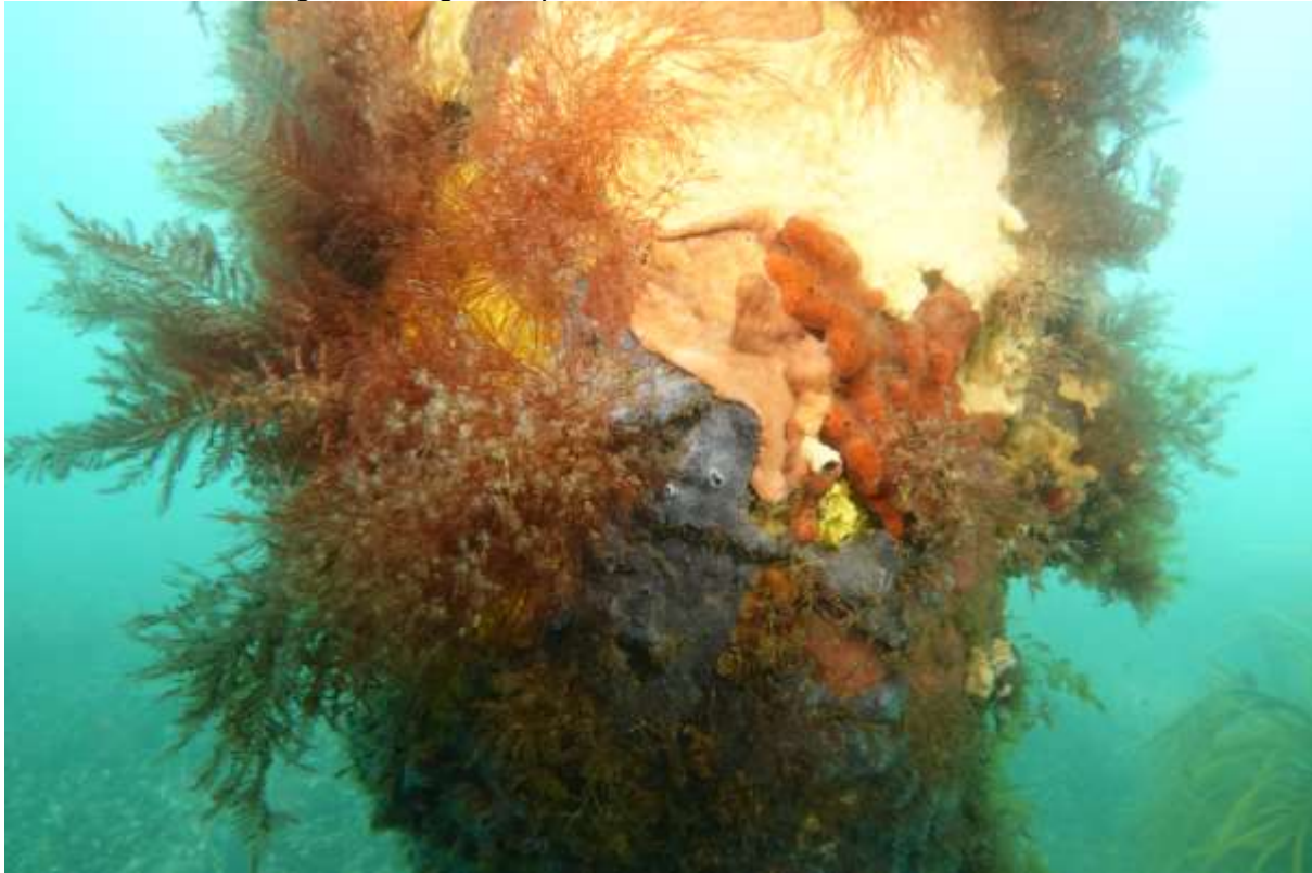
Attachment 30. Image showing steel pile 22F
