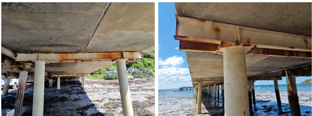
Figure 4-22: General condition of steel crossheads
